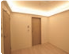
OLED lighting installed in residential unit at Sustainabranche Hongyotoku
