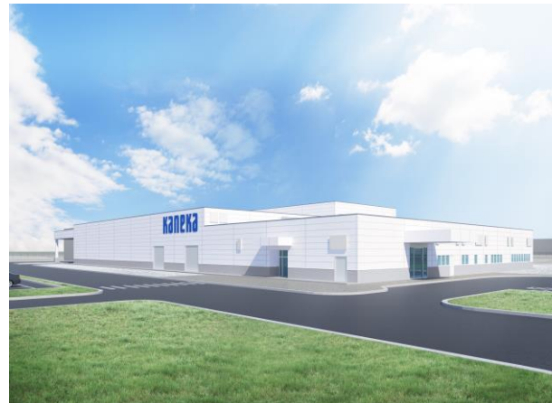
Medical Hokkaido Construction of a new production facility for blood purification devices
