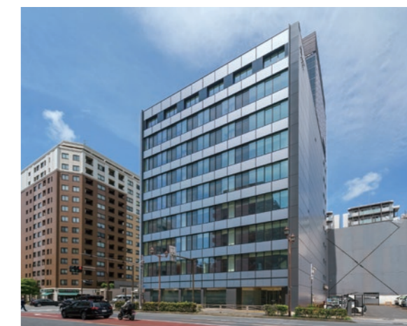
T-Green™ Multi Solar, a photovoltaic power generation system integrated with building external walls and windows, receives the Fiscal 2023 Minister of the Environment Award for Climate Action from Japan's Minister of the Environment
