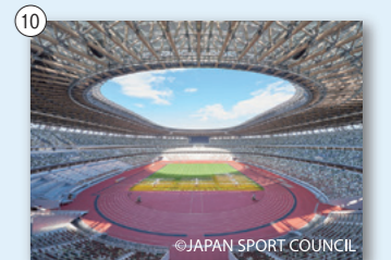
JAPAN NATIONAL STADIUM
